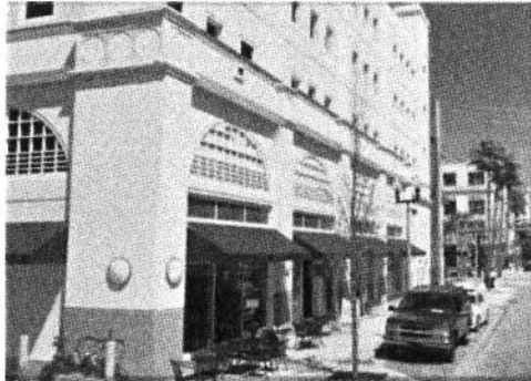
The Clematis Street garage utilizes consistent building materials with fenestration patterns to establish an attractive façade screening the parking levels over the retail space.
